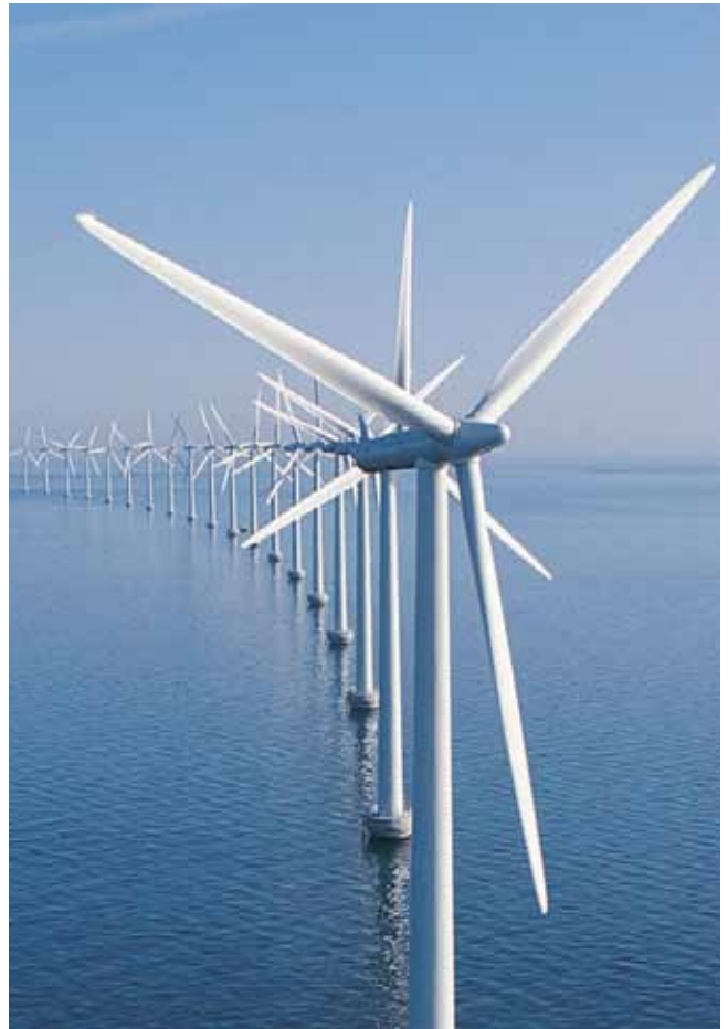
Offshore wind farm Thanet
